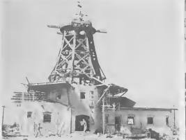
A NEW foundation, its architectural lines complimentary to the old mill's lines, supports the 147-year-old structure. UN FUNDESIO nobo, su lijnanan architectural complementando e lijnanan di e molina bieuw, ta wanta e estructura.
